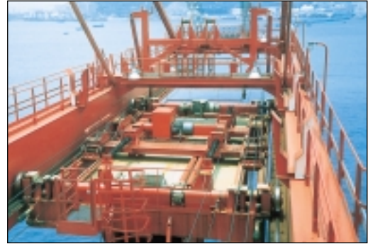
Anti Sway Mechanism, Ship to Shore Crane, Hong Kong.
