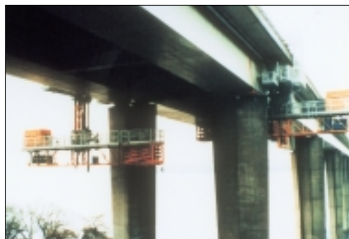
Inspection and Maintenance Platform, Tay Road Bridge.
